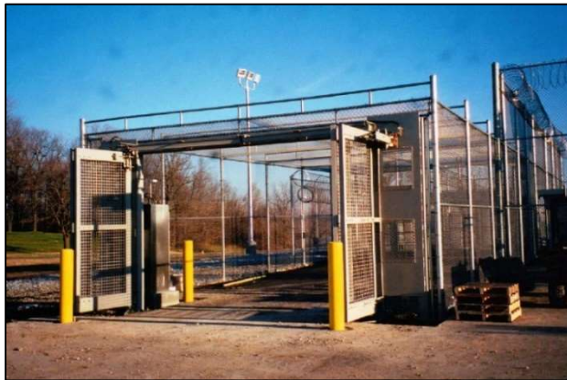
Figure 2: Sally port with cover - unrestricted area gates open / secure area gates closed.
