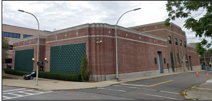
Figure 1: Neighborhood compatible substation
